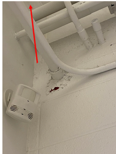
HM#1- Ceiling Concrete (Grey Painted White)
