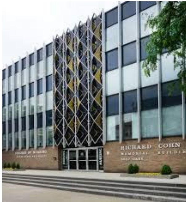
Richard Cohn Memorial Building 5557 Cass Avenue, Detroit, MI
