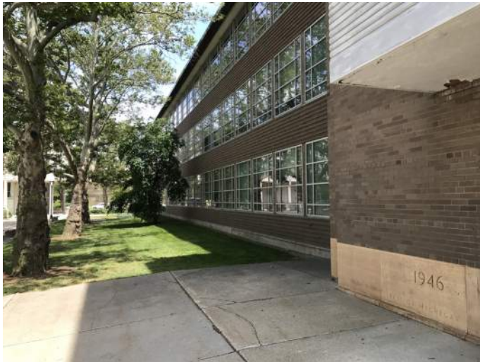
Figure 30: Existing State Hall West Facade
