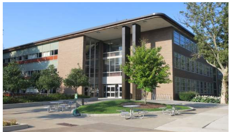
Figure 27: State Hall Cass Avenue Entrance
