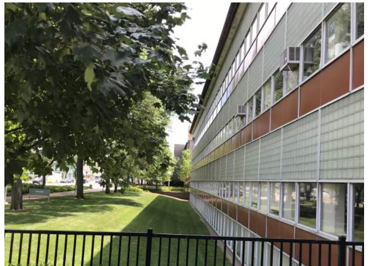
Figure 26: State Hall Cass Avenue Facade
