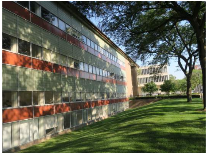
Figure 31: Existing State Hall North Entrance
