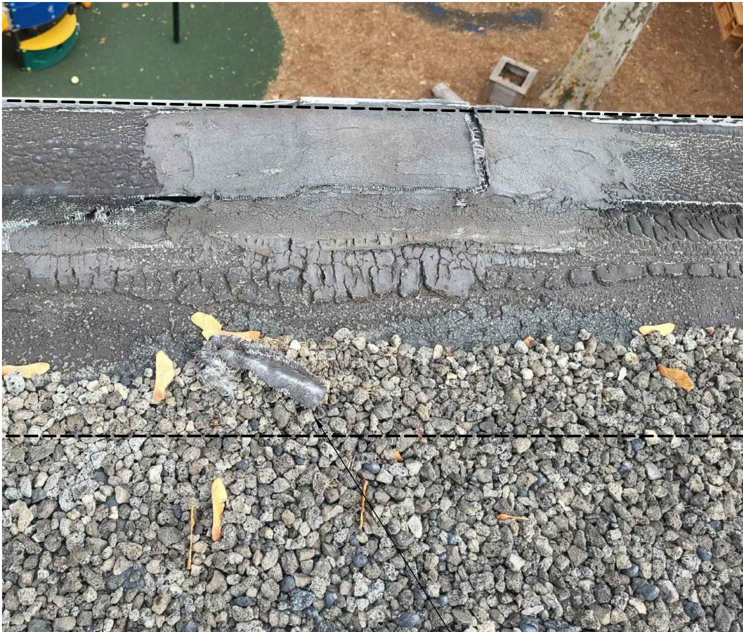
D13 A-502 TYPICAL PORCELAIN ENAMEL PANEL FLASHING REPLACEMENT - LOWER
