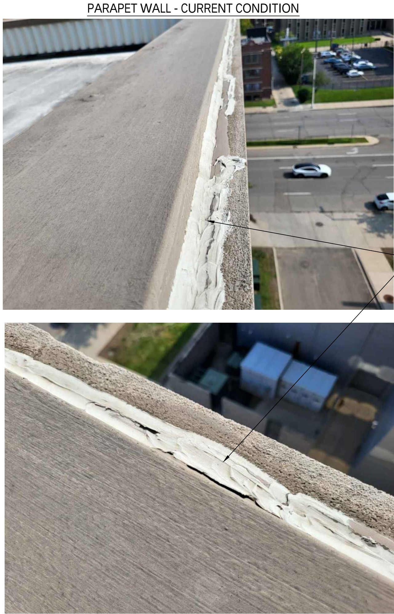
SEALANT REPLACEMENT AT PARAPET WALL
