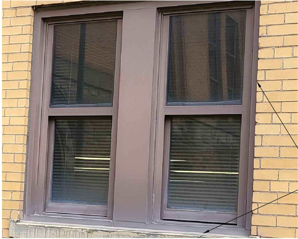
TYPICAL WINDOW SEALANT JOINT REPLACEMENT
