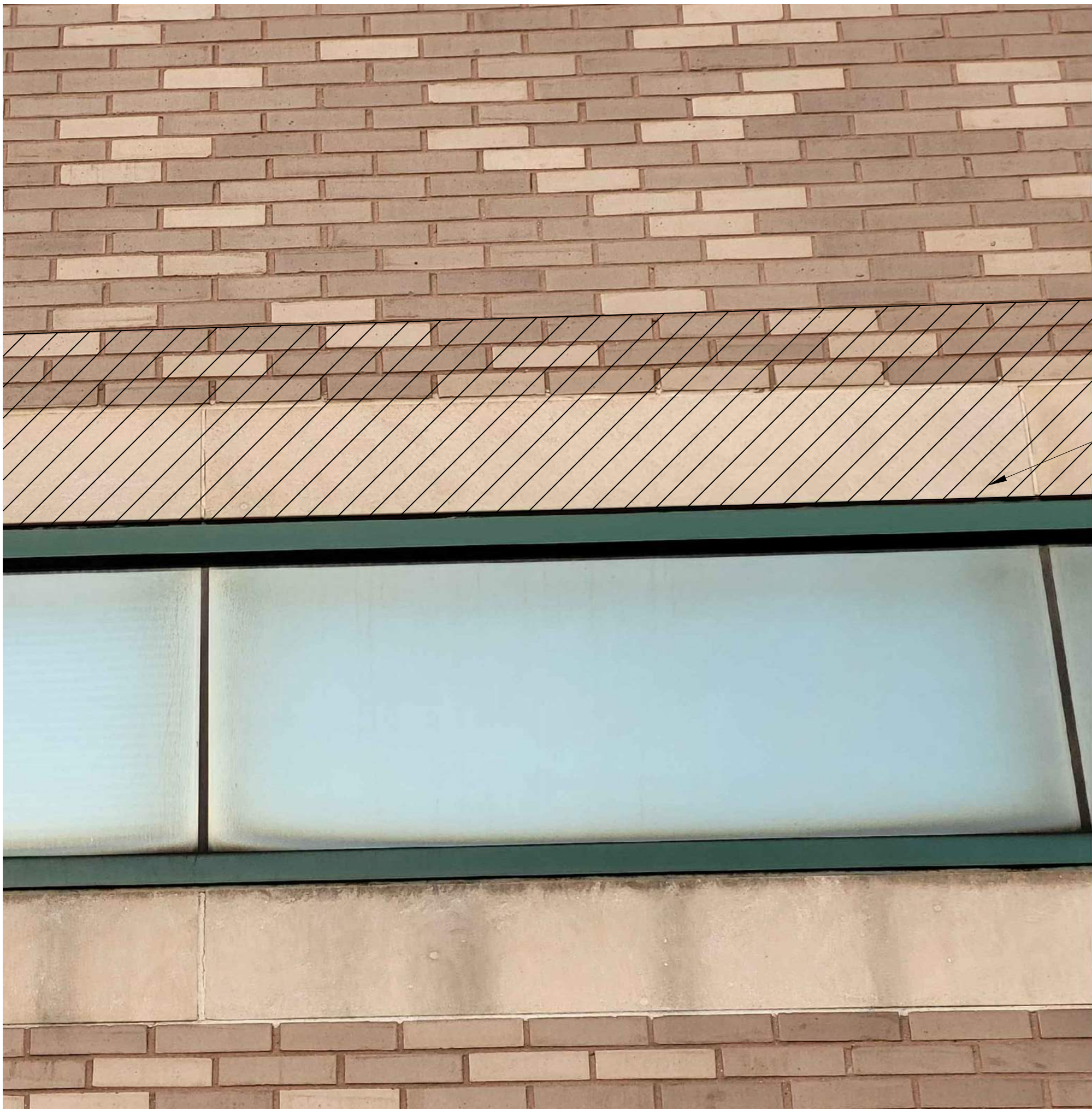
TYPICAL THROUGH WALL FLASHING/LINTEL REPLACEMENT DETAIL - LIMESTONE
