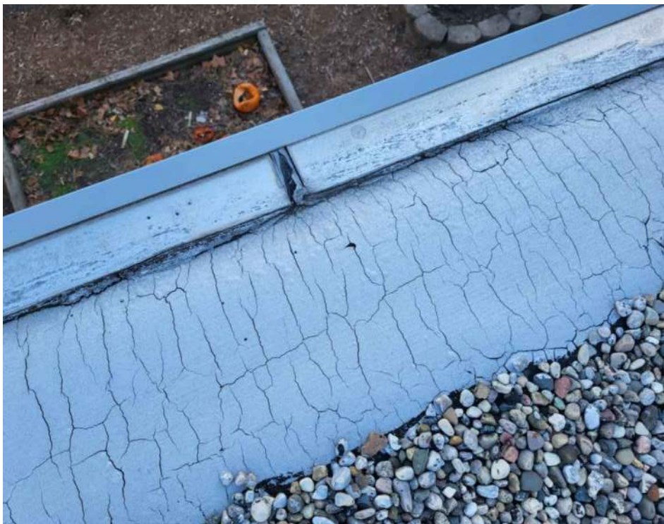
CURRENT CONDITION - PERIMETER OF ROOF B
