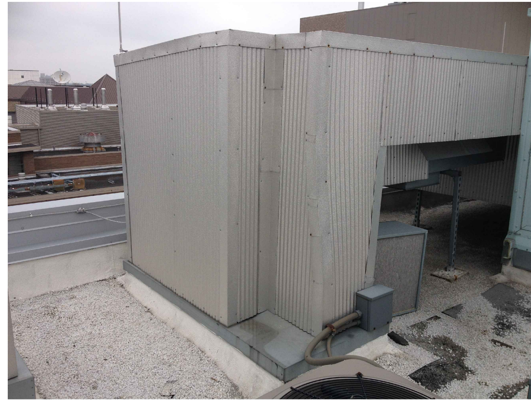
PHOTO 1 - EXISTING ENGINE EXHAUST DUCT ENCLOSURE NO SCALE
