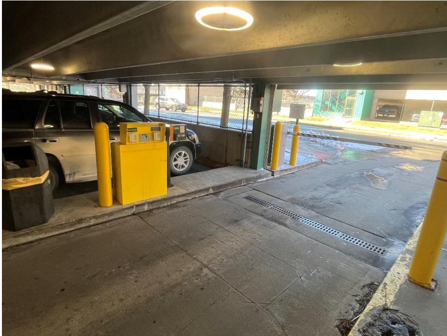
Photo 41: Parking Structure 2 – Gate 1
