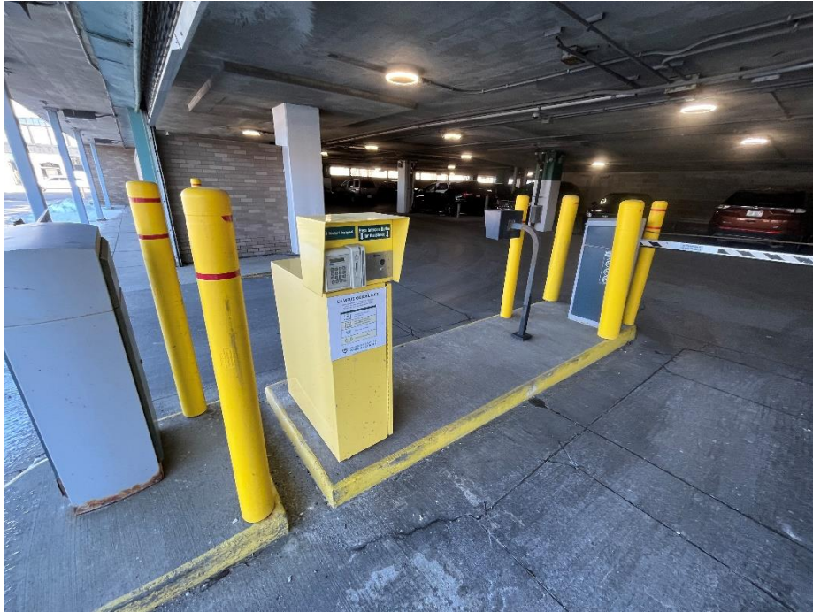
Photo 35: Parking Structure 1 – Gate 1
