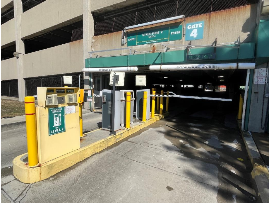
Photo 43: Parking Structure 2 – Gate 4
