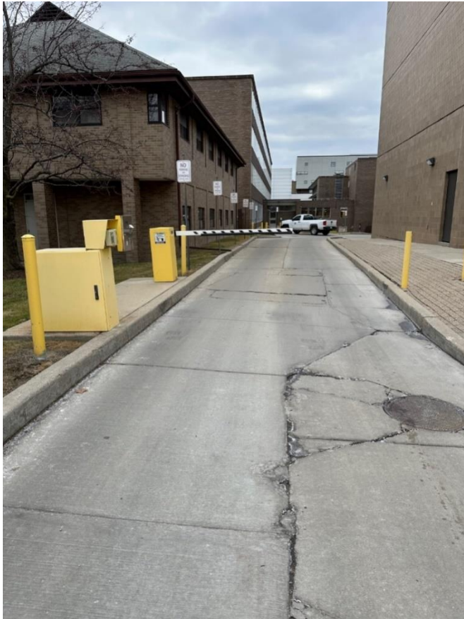
Photo 69: Rands/Purdy Library Loading Dock
