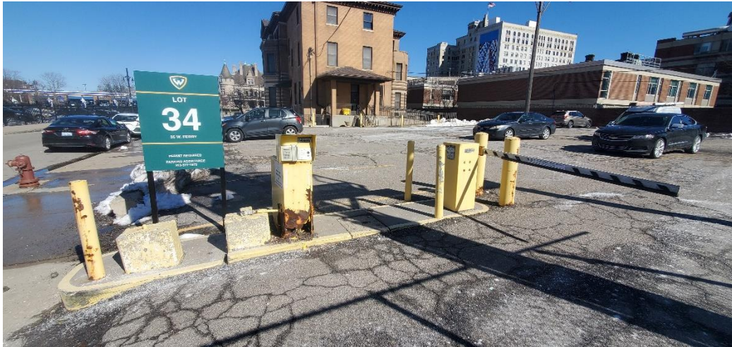
Photo 14: Lot 34 (See Exhibit A for requested changes at this location)
