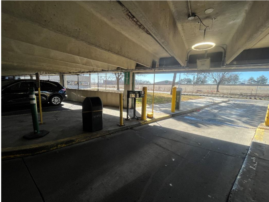
Photo 45: Parking Structure 2 – Gate 6
