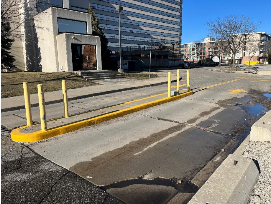
Photo 31: Lot 72 (this lane is not used now or planned for the future)
