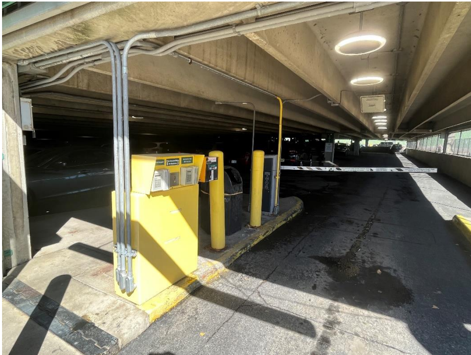
Photo 42: Parking Structure 2 – Gate 3
